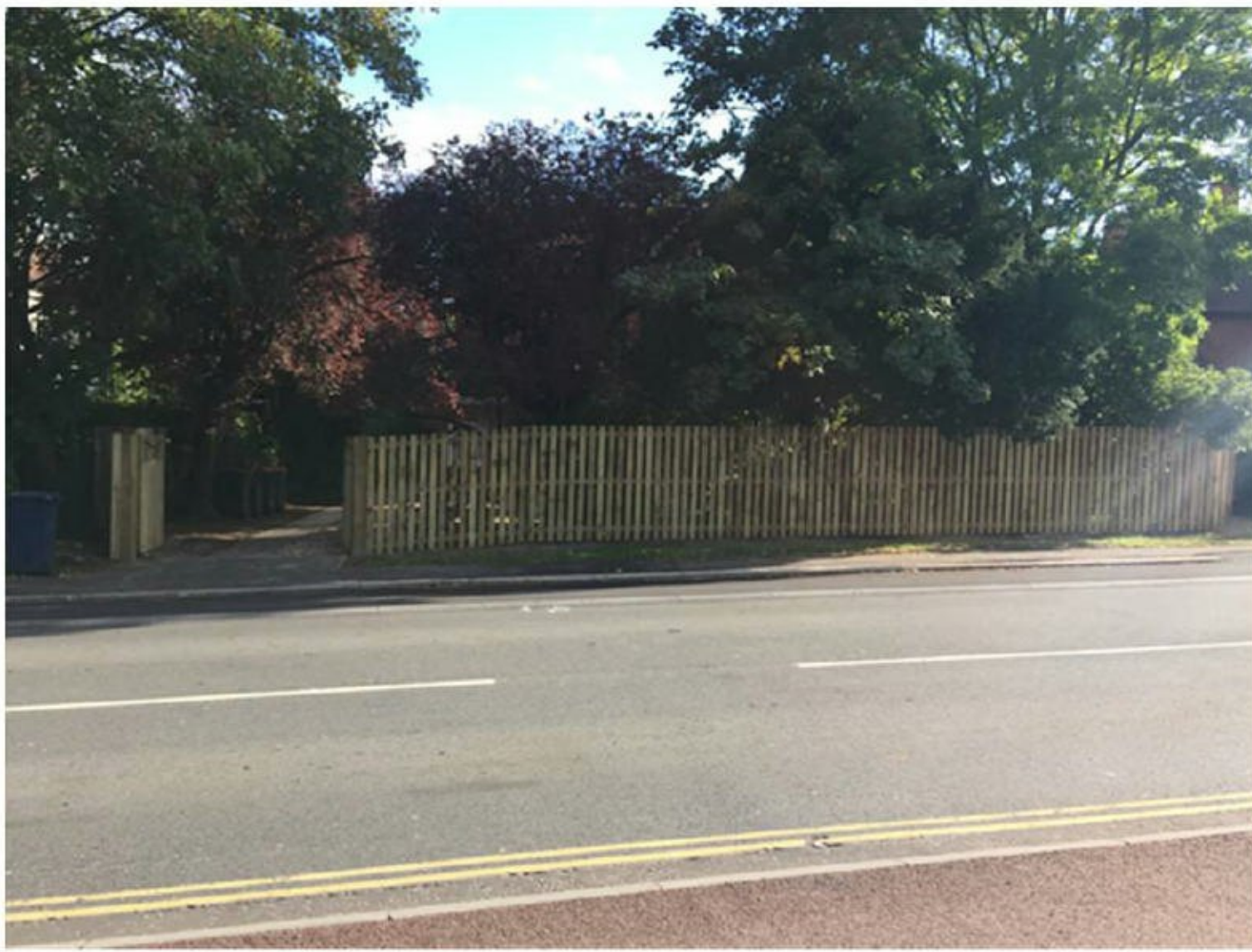
Picture 1 – Fence and gate installed at 285 and 287
