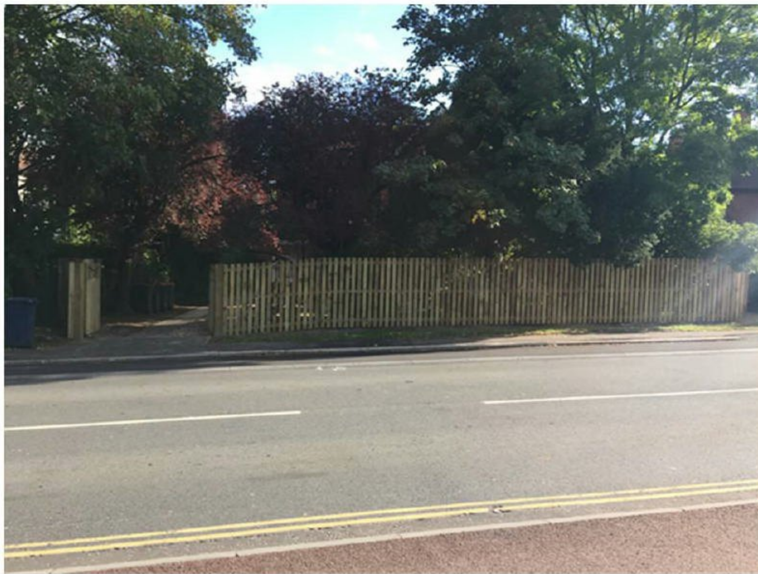
Picture 1 – Fence and gate installed at 285 and 287
