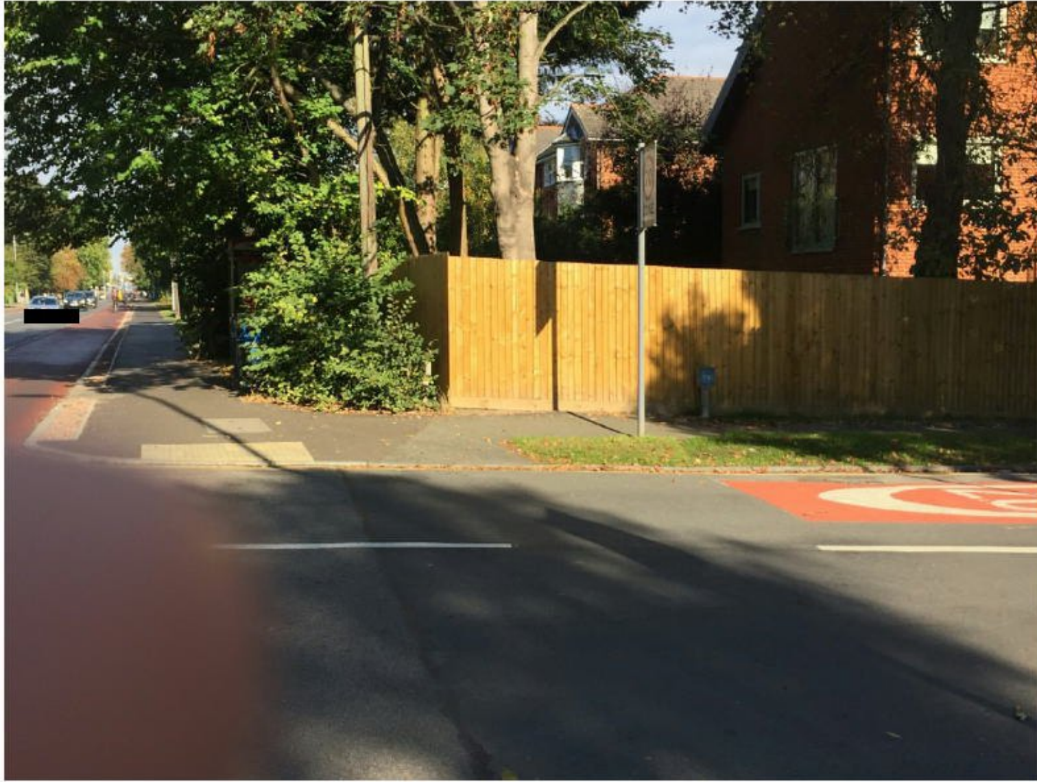
Picture 4 – Fence along Hills Road
