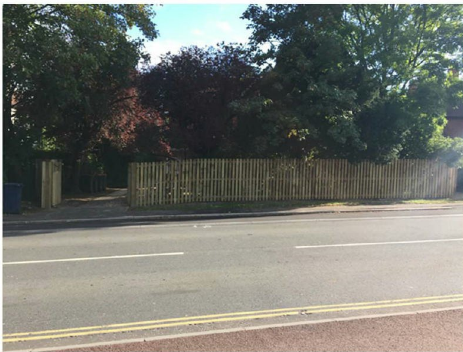
Picture 1 – Fence and gate installed at 285 and 287
